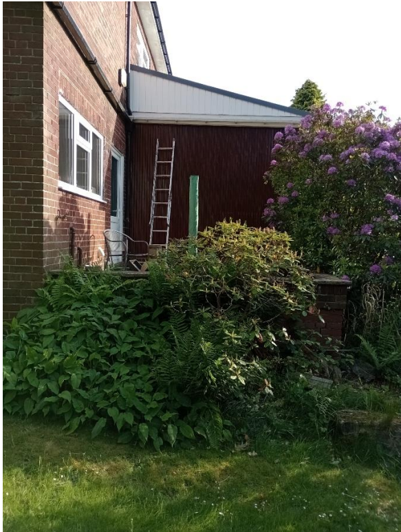
Wall where door will be added
