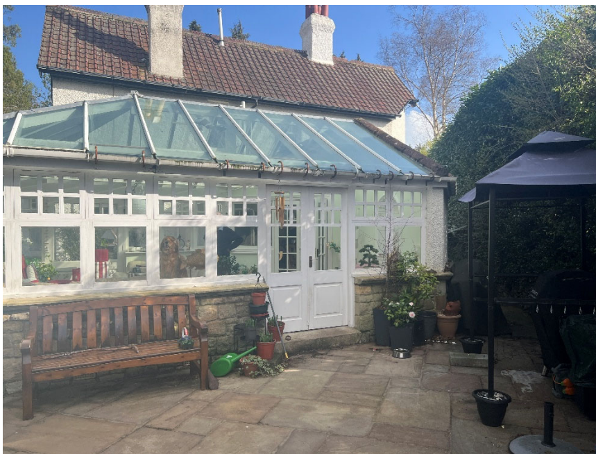
Figure 12: Existing rear sun room
