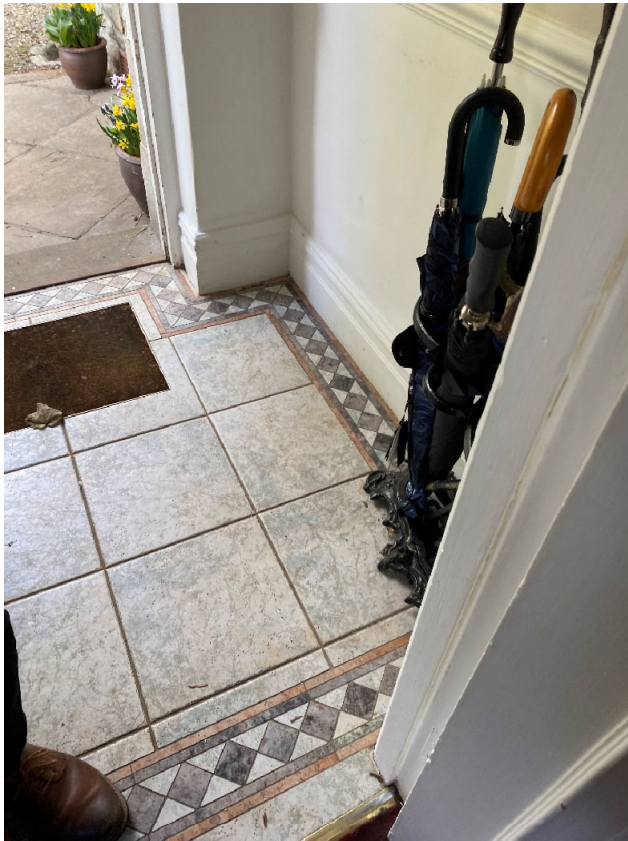
Figure 8: Existing interior of entrance lobby
